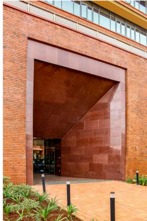
JHANSI RED GRANITE ON MAGNETIC CLADDING
