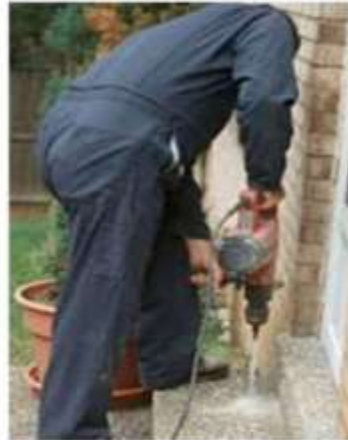
PREPARING HOLE FOR TERMITE PURPOSES
