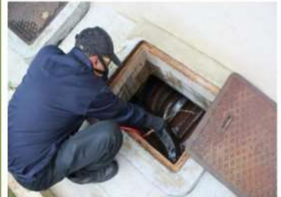
SPRAYING CHEMICAL FOR DRAINAGE SYSTEM
